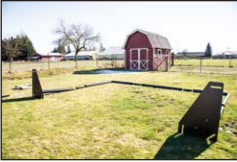
Photo1 - Tilt base to remove sod
