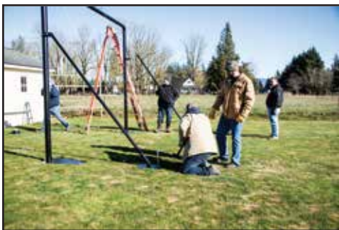
Photo 4- Standing up the end frame
