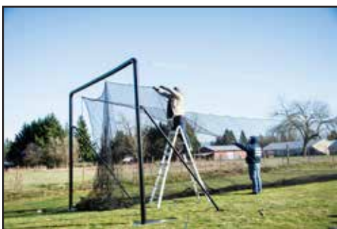
Photo 5- Attach carabiners onto cables
