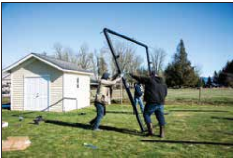
Photo 4- Standing up the end frame
